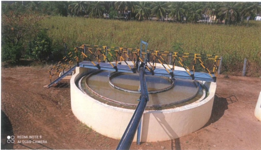
Figure 6 :Clariflocculator
